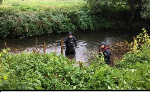
The Environment Agency's Ben Norrington and Andy Ward worked tirelessly on both days installing the features on the river .
