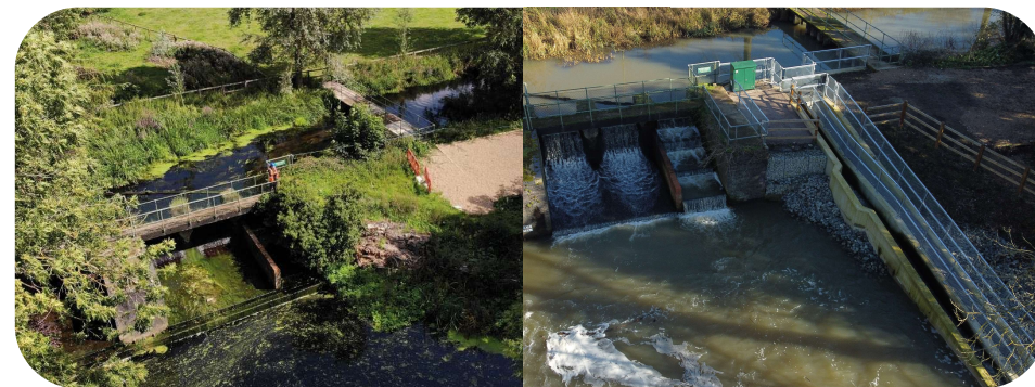
Langford weir, upstream of the Museum of Power, before and after the installation of a new fish pass during 2024/5. This structure opens up the river between Beeleigh and Wickham Bishops and serves as an example of a type of fish pass project that could be completed elsewhere on the Pant and Blackwater. Photos provided by principle contractor; Stonbury
