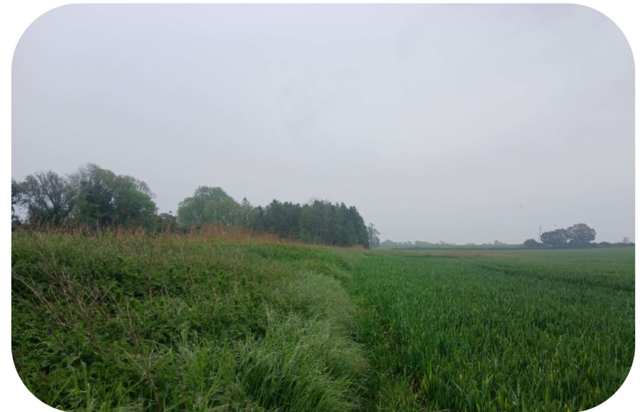
Embankment along this reach of the Pant. The embankment is around 1-2m high compared to the floodplain. The Pant is not visible here due to the embankment and incised channelling, but in places the channel is around 3m deep or more.
