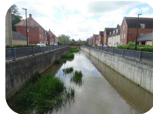
The Blackwater at Bocking, view looking upstream towards the Pant. Despite high flows, it is possible to see where silt deposits have created a sinuous river channel
