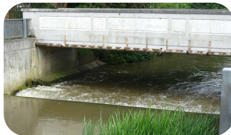
Looking downstream from the same point, a weir can be seen, one of a number throughout the catchment that could be considered for modifications for improved fish passage
