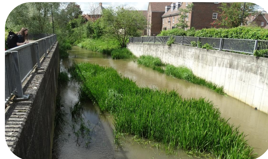
Surveyors overlook the point where the Pant becomes the Blackwater at Bocking, Braintree. At this site, the overwide river has deposited silt which has allowed vegetation to build up, creating a more sinuous, natural channel within the larger concrete channel. The site now attracts wildlife including nesting swans
